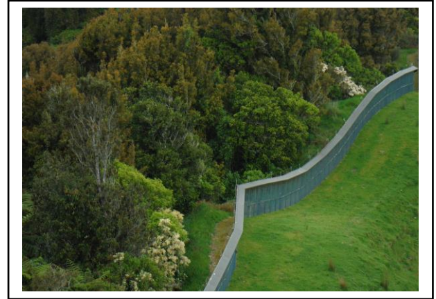
Fence hood, mouldy areas need a clean this month
